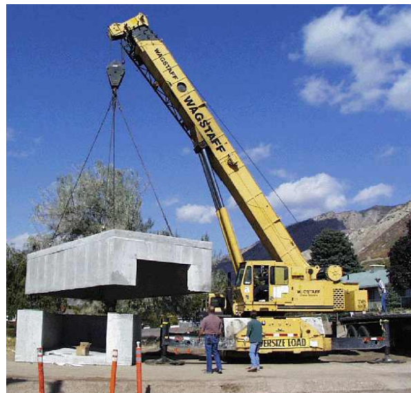
Figure 4. The crane is fitting the top half of the observatory to the bottom half. There is a tar sealing strip in between the two halves.
