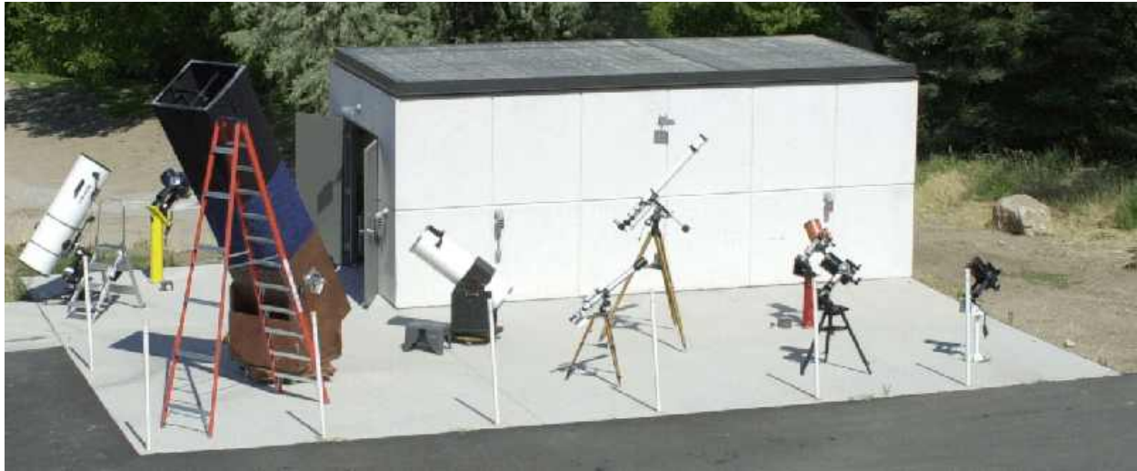
Figure 1. Department of Physics Observatory, the building dimensions are 12 feet X 24 feet X 10.5 feet (3.6m X 7.3m X 3.2m) (W X L X H). Notice the red lights on the exterior.
