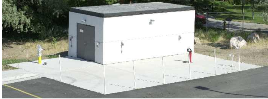
Figure 5. The finished observatory building, phase I.
