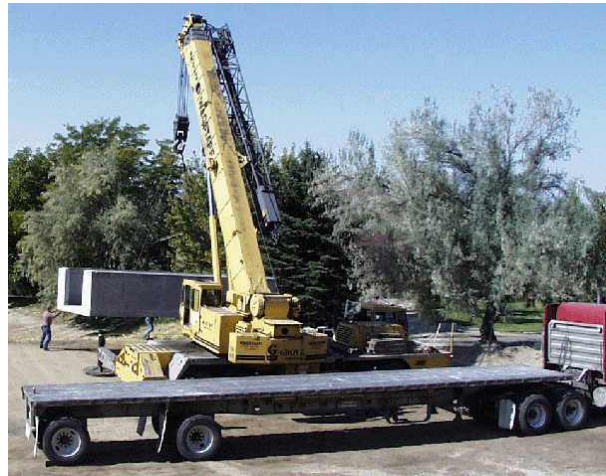
Figure 3. Setting the base half on the prepared ground.
