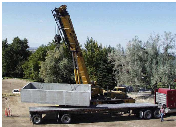
Figure 2. Removing the base half from the flatbed truck.
